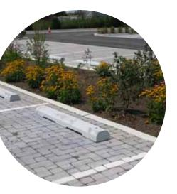
Example of a parking lot stormwater BMP with permeable pavers and an integrated vegetated swale.
